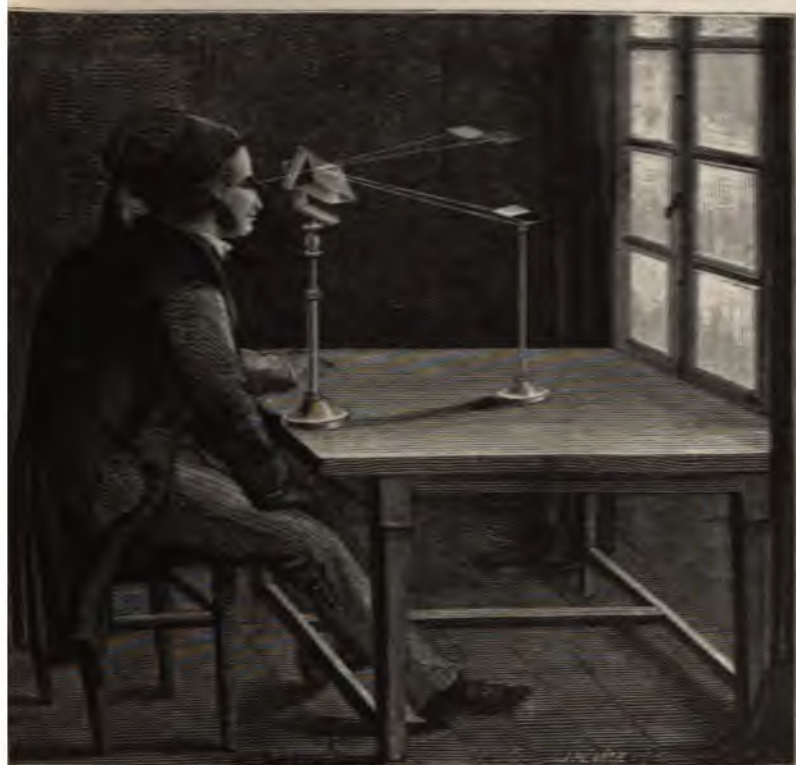
FIG. 39.—Unequal refrangibility of two differently coloured lights.
